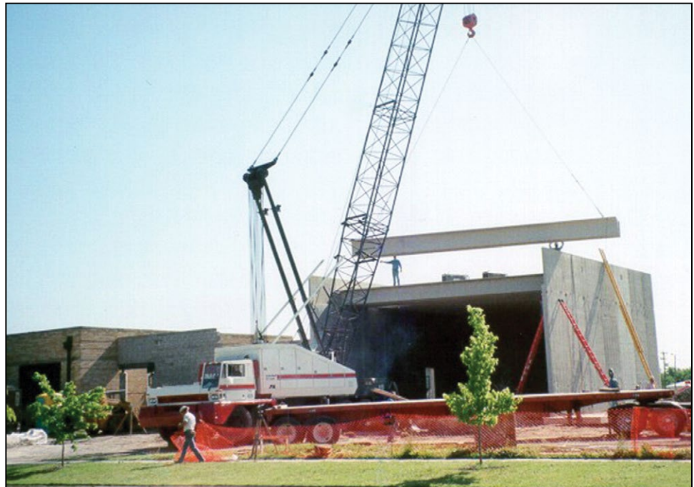
Figure B1-1. The addition to this school was designed to serve as a multi-use safe room; it is also used as a cafeteria, gym, and for large group gatherings (Wichita, KS)
